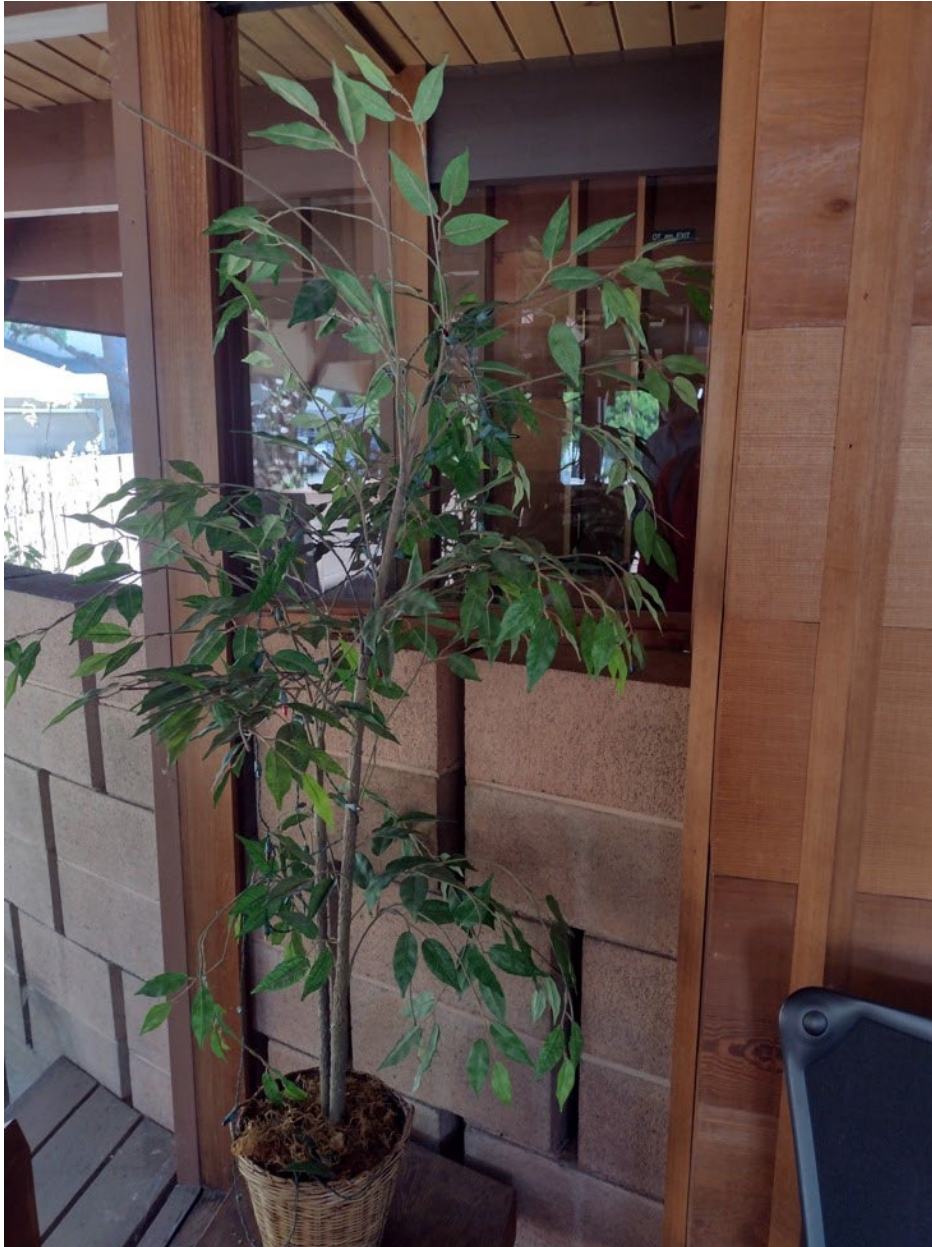
Photo 8. Exterior concrete block fence intersecting with glass wall
