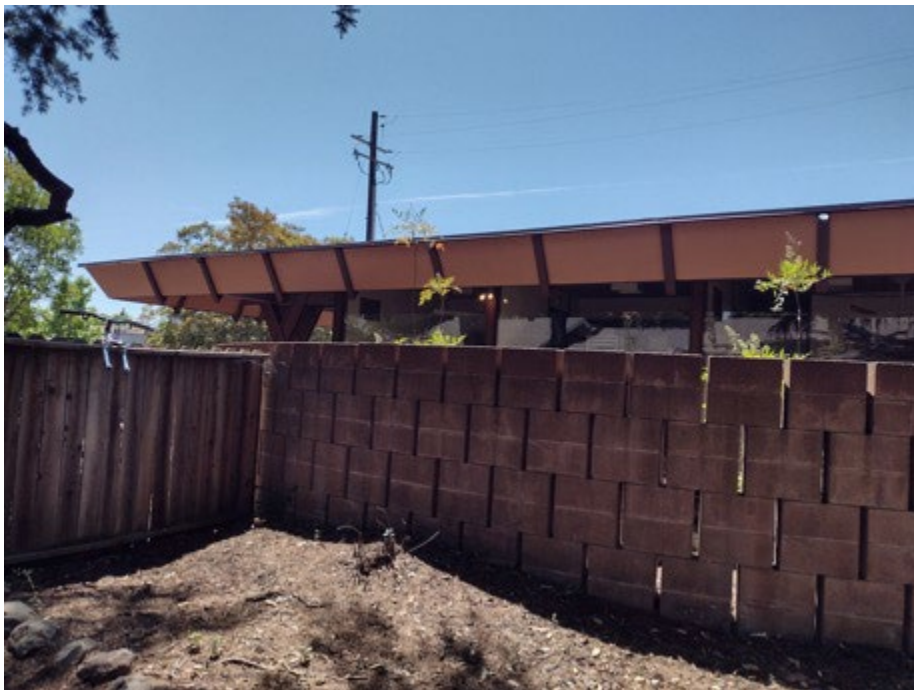
Photo 5. West/Rear elevation, South bay (GA, 2025)
